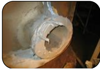
Flange face reforming using 101 Power Metal Repair Paste
