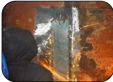
Corroded gas tank holder repaired using PES 106 Power Metal Repair Paste XF
