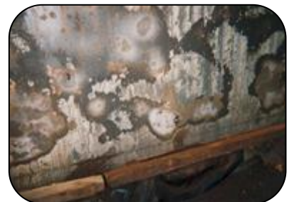
Corroded gas tank holder repaired using PES 106 Power Metal Repair Paste XF
