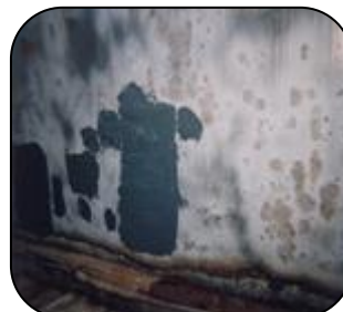
Corroded gas tank holder repaired using PES 106 Power Metal Repair Paste XF
