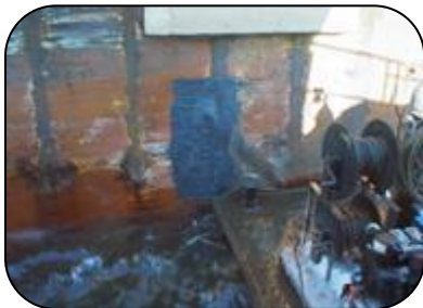
Holed ship hull repaired in sub-zero temperatures using PES 106 Power Metal Repair Paste XF and a formed steel plate
