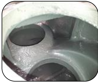
Sea water filter operating at 203°F (95°C) coated with PES 205 Ceramic HT Fluid
