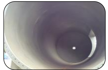
Paper plant chimney operating at 212°F (100°C) with traces of sulphuric acid coated with PES 206 Ceramic HTA Fluid
