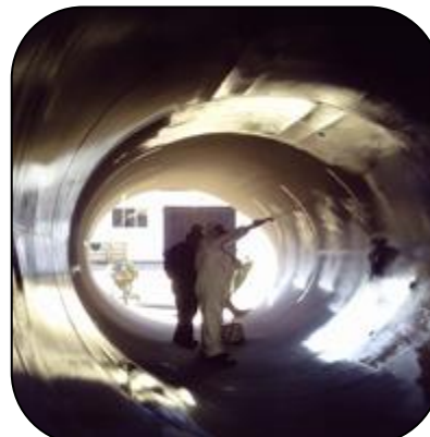
Paper plant chimney operating at 212°F (100°C) with traces of sulphuric acid coated with PES 206 Ceramic HTA Fluid
