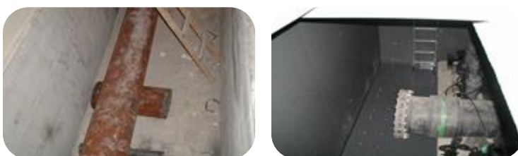
Chemical pit coated with PES-Chem 511 UCEN
