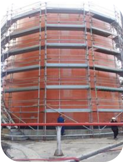
Oil storage tank, water jetted at 500psi and coated with PES-Chem 555 Pesinox – 10 mils stripe coat with 2 coats at 14 Mils WFT
