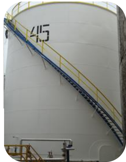
Oil storage tank, abrasive blast cleaned to Nace 2 near-white blast with 3-4 mil profile. Stripe coated with 10 mils of PES-Chem 501 CRSG, 1 x coat of PES-Chem 501 CRSG applied by standard airless spray at 12mils WFT, 1 coat of PES-Chem 508 UVPU applied by standard airless spray at 5 mils WFT
