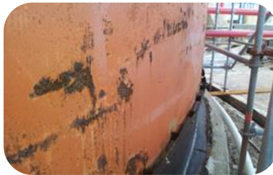
Oil storage tank, water jetted at 500psi and coated with PES-Chem 555 Pesinox – 10 mils stripe coat with 2 coats at 14 Mils WFT
