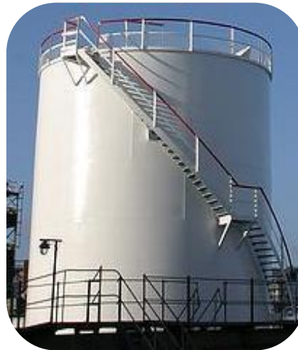
Oil storage tank, water jetted at 500psi and coated with PES-Chem 555 Pesinox – 10 mils stripe coat with 2 coats at 14 Mils WFT
