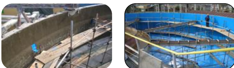
Concrete river water tank coated with PES-Chem 501 CRSG
