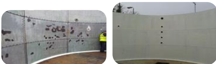
Sectional steel tank coated with PES-Chem 507 DWPU
