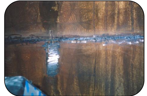
Damaged tank seams filled and rebuilt using PES 102 Power Metal Repair Fluid
