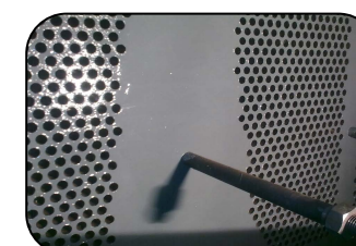
Condenser tube sheet resurfaced
